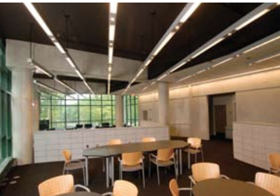
The interior of the Overlook consists of unfinished precast concrete, which reduces the need for maintenance a great deal and provided the college with value engineering.
